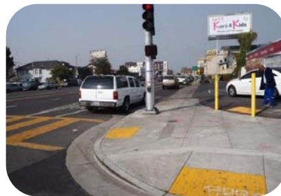
ADA ramp upgrades
