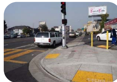
ADA ramp and signal upgrades
